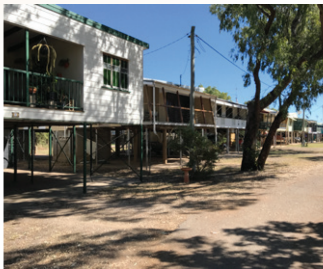
Groper Creek elevated dwellings
